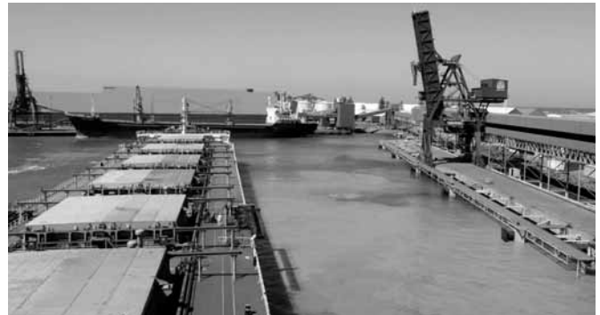
Loaded Panamax Pulling off berth 5
